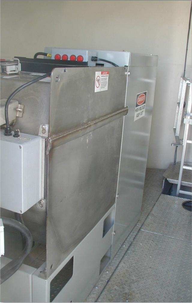
*Inside of one-way Vista switchgear unit
