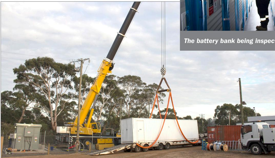
*Crews install the containerized PureWave® SMS Storage Management System.*
