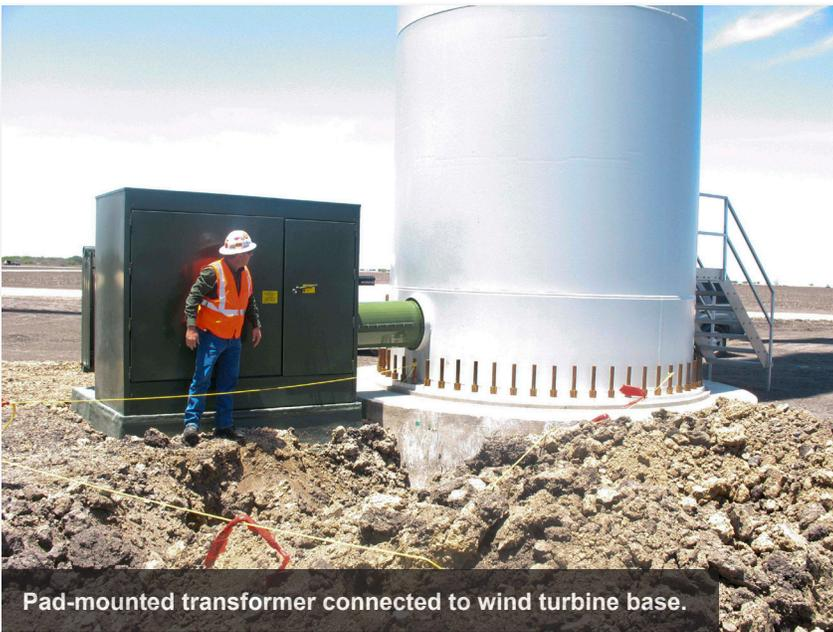
Pad-mounted transformer connected to wind turbine base.
