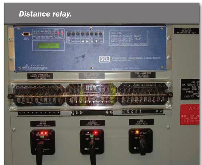
chargers, protective relays, and auxiliary devices, all the way to dual trip coils on the circuit breakers. Redundant differential relaying is used, featuring relays from different manufacturers. Each differential relay reverts to a back-up distance relay scheme if communication is interrupted.
